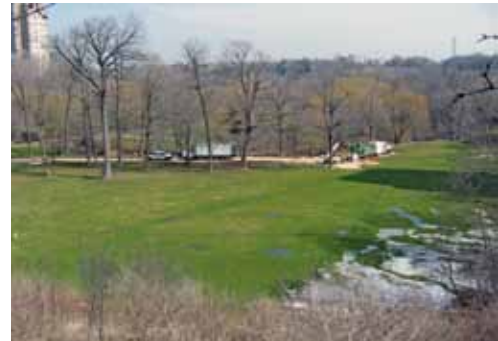
The rehabilitated pipe and culvert carry storm water through a golf course.
