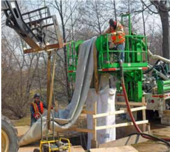
Host pipe was up to 48 inches (1,219 millimeters) in diameter.
